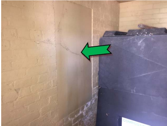
Photo 7. Interior, lower ground, toilet, tank room, western wall – non asbestos-containing fibre cement sheeting.
