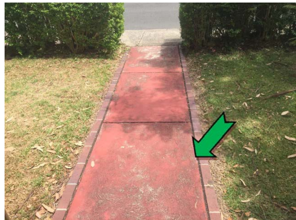
Photo 4. Exterior, west elevation, foot path – non asbestos-containing bituminous material.
