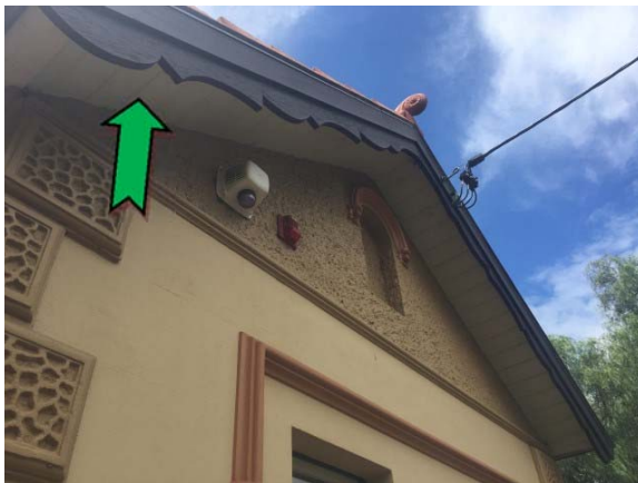
Photo 3. Exterior, throughout, eaves – suspected non asbestos-containing material.
