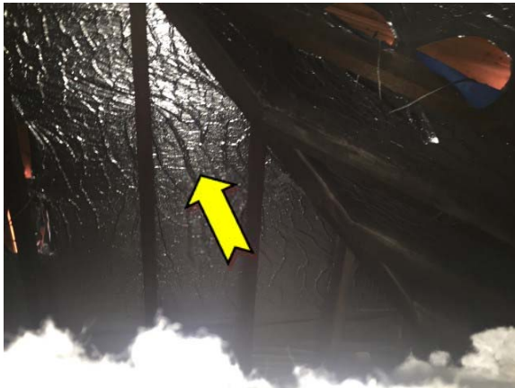
Photo 9. Interior, ground level, throughout, ceiling space – suspected SMF sarking insulation .
